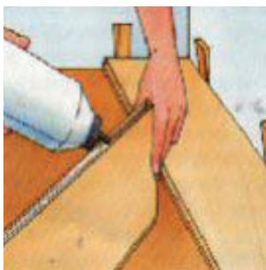
The correct order to lay the boards is shown above 1-6. Now dismantle and re-assemble the boards in the same sequence, this time gluing the boards together.
