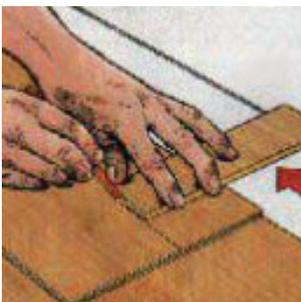
The last row of planks will need to be sawn lengthwise. Lay the last plank directly over the last but one board. Then using an off-cut board scribe a cutting line down the board.
