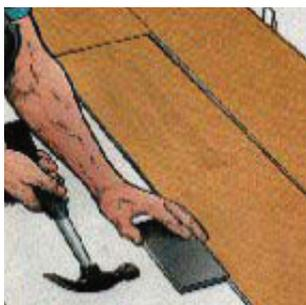
Use a nylon or beech tapping block to lightly knock in the second row of boards. It is important to always hit the tongue and not the edges of the boards
