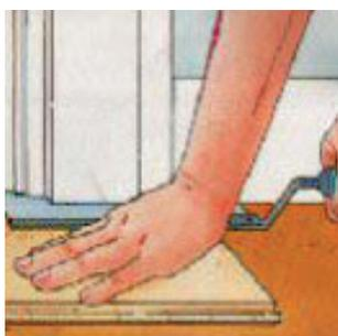
Cut through architraves and door casings with an under cut saw using an off-cut board as a guide. The floor can then be slid under making a neat finish.
