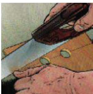
Cut through the holes as neatly as possible. It may help to first cut through the surface of the board with a stanley knife.
