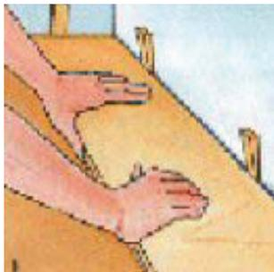
Lay groove side to the wall, using spacers to maintain a 10 mm expansion gap between the boards and the wall. Do not apply any adhesive at this stage.
