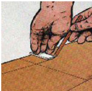
If the wall runs out, lay the boards straight to the chalk or laser line a few cms from the wall and scribe a straight line with a pencil. Cut down the board to line up with the wall, but insert spacers.
