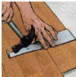
Apply glue to the groove and the pull the board into place with the pulling iron. Ensure that the board is held tightly by inserting spacers.
